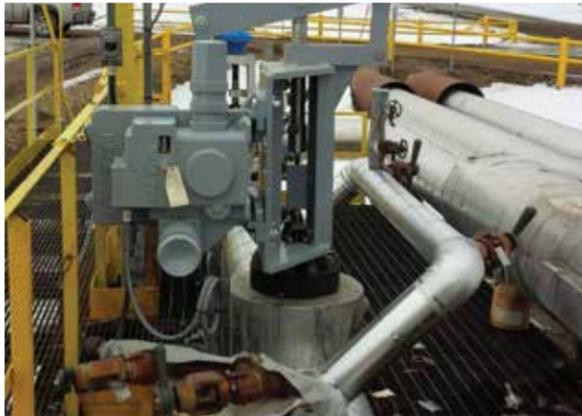
Figure 3. Actuator and fulcrum lever mounting assembly.
