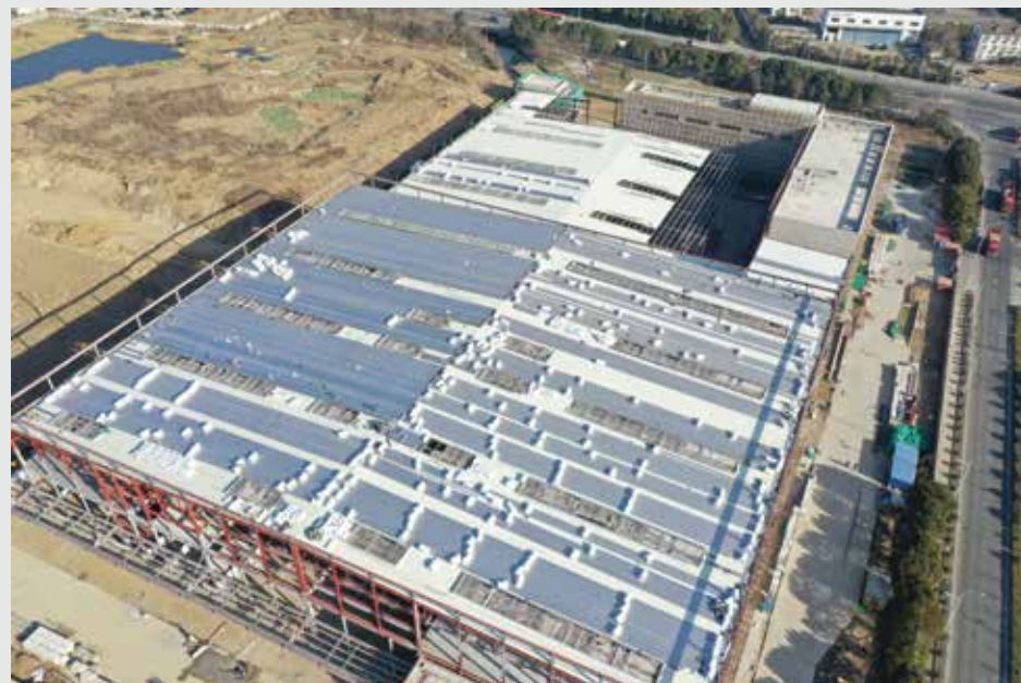
67000sqm New Butterfly Assembly Plant (Estimated Operation Date: 2021 Q4).
