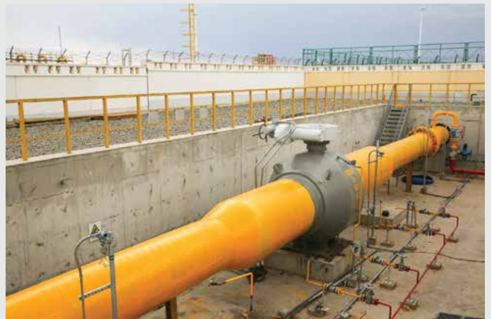
56" Full Welded Ball Valve.
