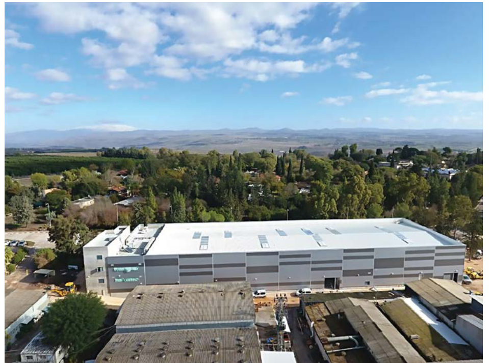
Overhead view of new production in facility in Israel
