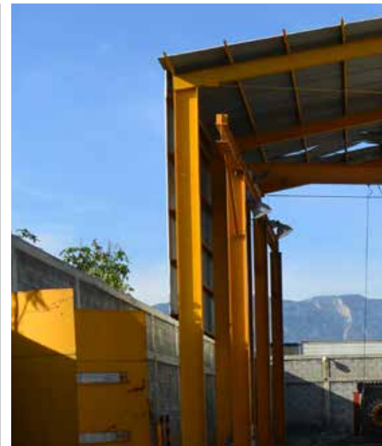
BS&B High Volume, Set Pressure Testing Facility
