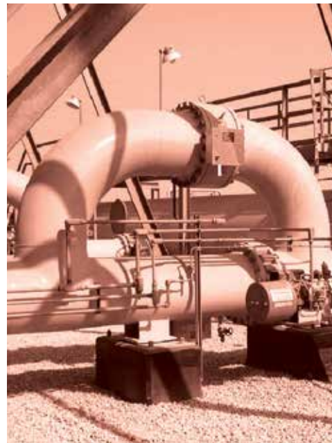
BPRV™ installed as inline bypass to staging valve on a gas flare system
