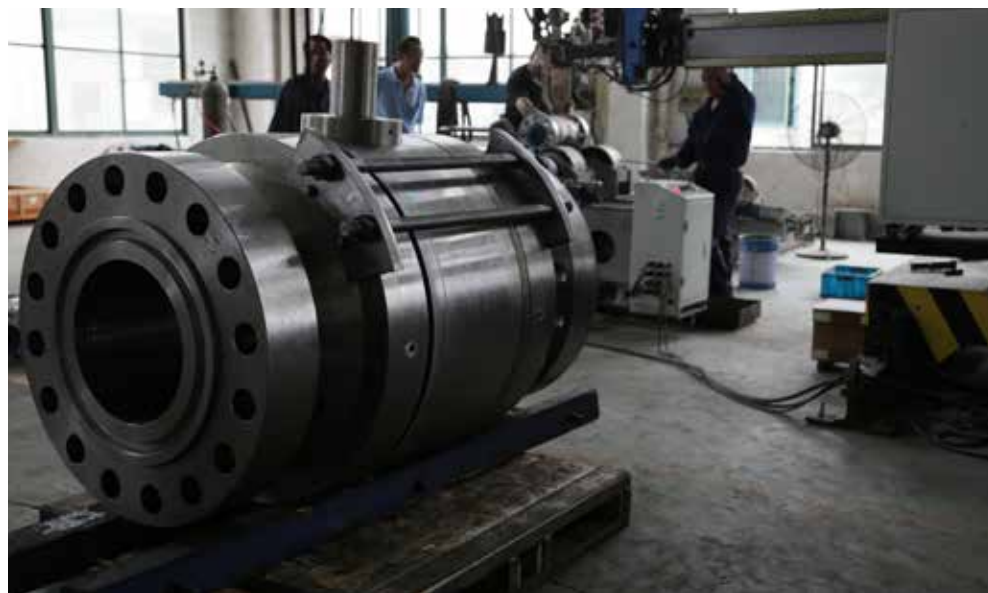
Fully Welded Ball Valve with Special Jig before Welding
