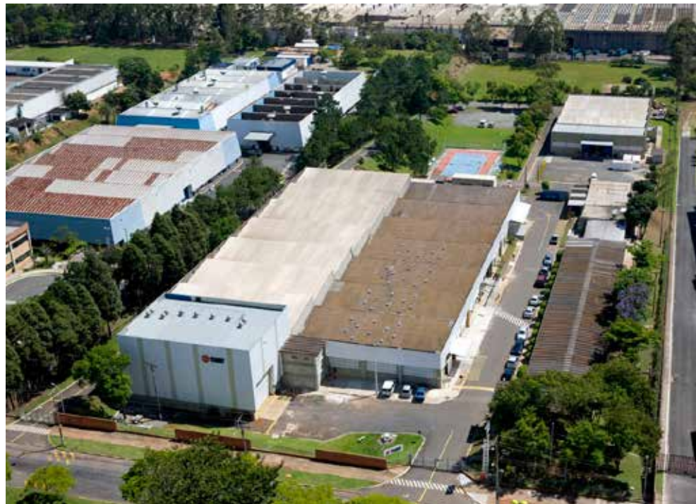
Teadit's main research and development plant located in Rio de Janeiro, Brazil
