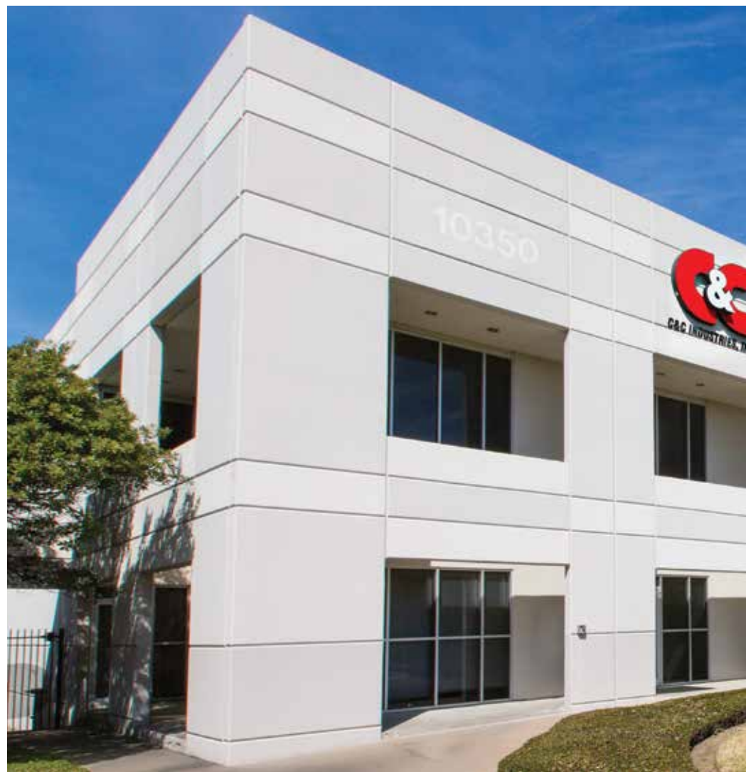
C&C Headquarters – Located in Houston, Texas.
