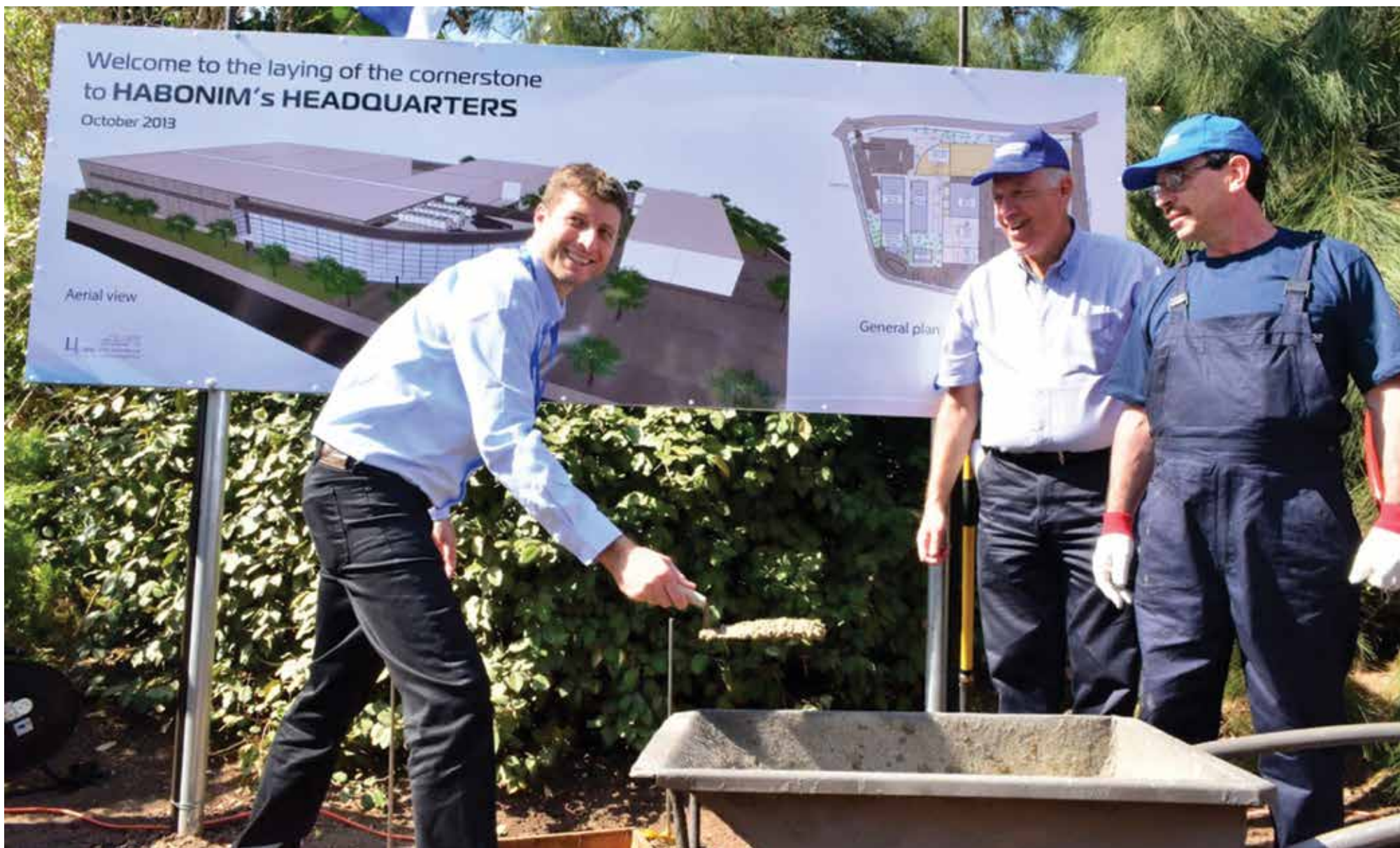
CEO Mr. Eliad Katz laying the cornerstone of the new Habonim house
