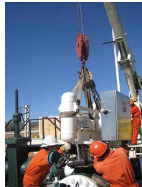
Workers install a Twin Power range pipeline actuator in Mexico.
