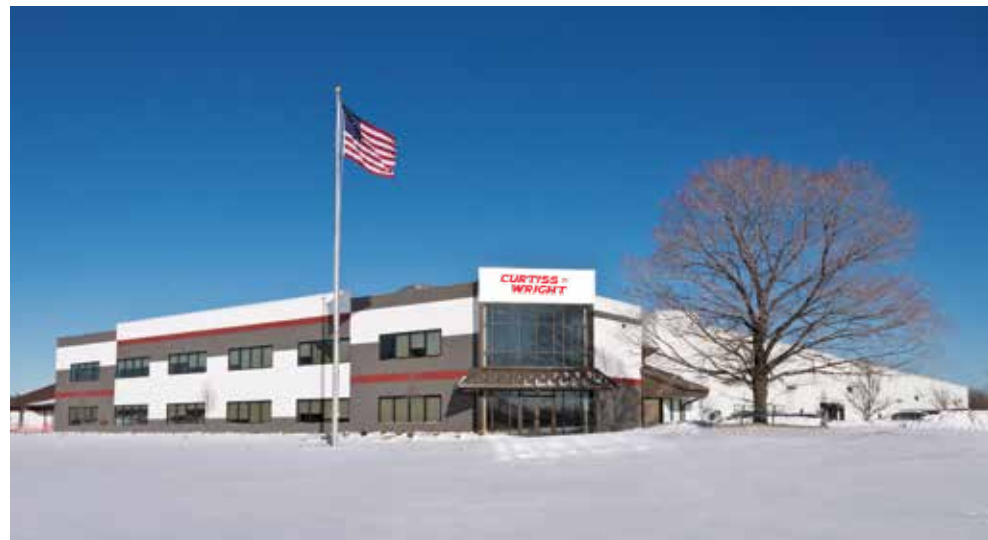
Farris Engineering's headquarters located in Brecksville, OH.
